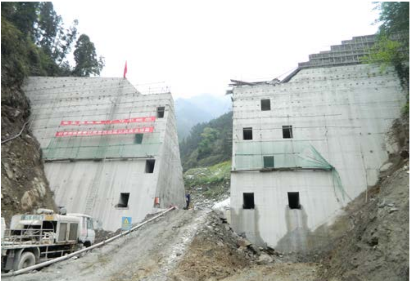
Debris flow dam in Zhangjiaping Village, built in 2014 to protect the village during heavy rainfall. Photo: Yingxiu Town government
