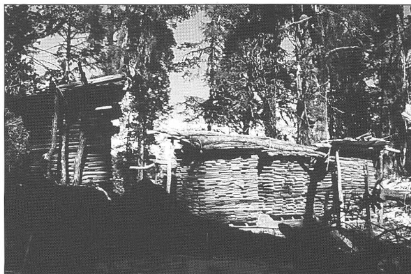
Roofing shingles cut from high altitude forest, Nepal
