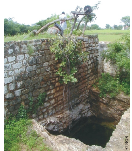
Prior to mechanised pumps, water was lifted from wells by mhots - large leather pouches pulled by cattle
