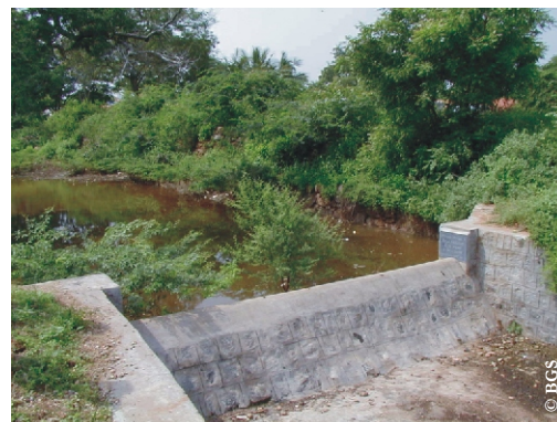
A small check dam in Coimbatore District
