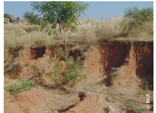
Excavation to provide storage upstream of a check dam. Households are paid by the volume of material removed: small earth walls show the boundaries between where different households have been digging.
