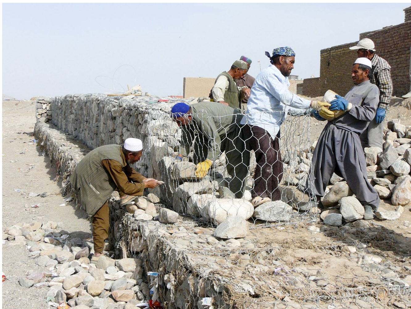
Men on the banks of the Harirod River in Herat, Afghanistan build a retaining wall to limit flooding. Photo credit: UNOPS, 2011.
